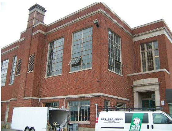
Main building (365A), south (rear) elevation at boiler room, looking northwest.
