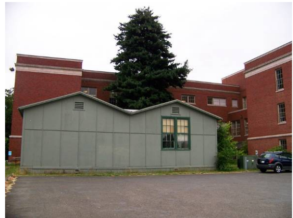
Main building (365A) and Portable (365P5), south (rear) elevation, looking north.
