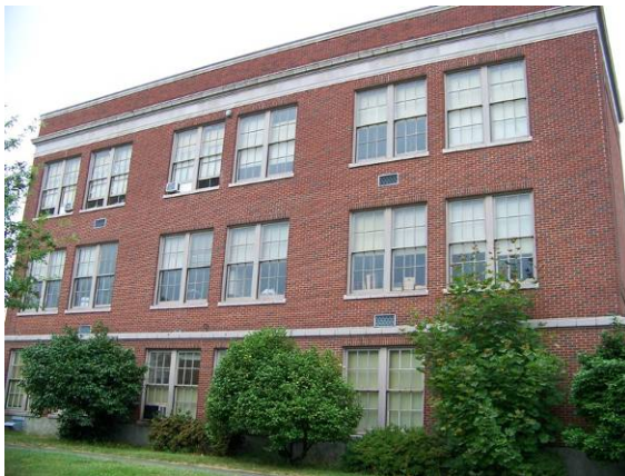
Main building (365A), east (side) elevation, looking west.
