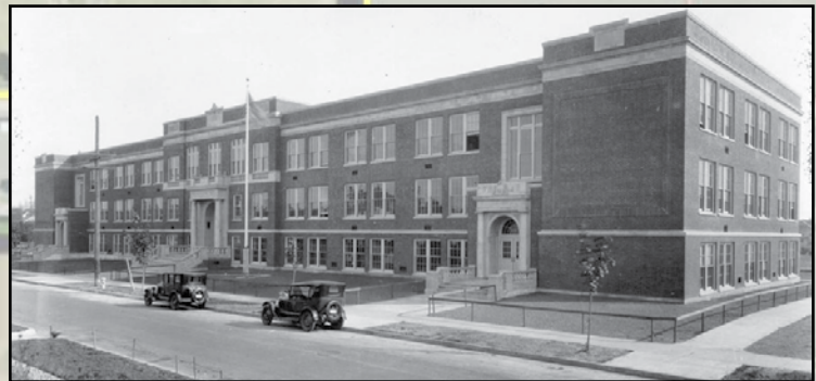
Late 1920s photograph of the Girls Polytechnic School (now Da Vinci School), looking south.
