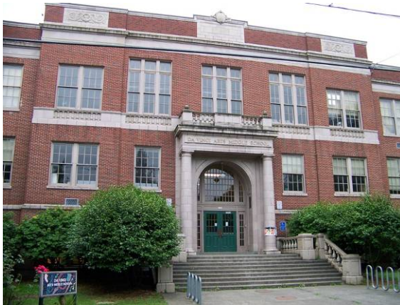
Main building (365A), north (front) elevation, looking south.
